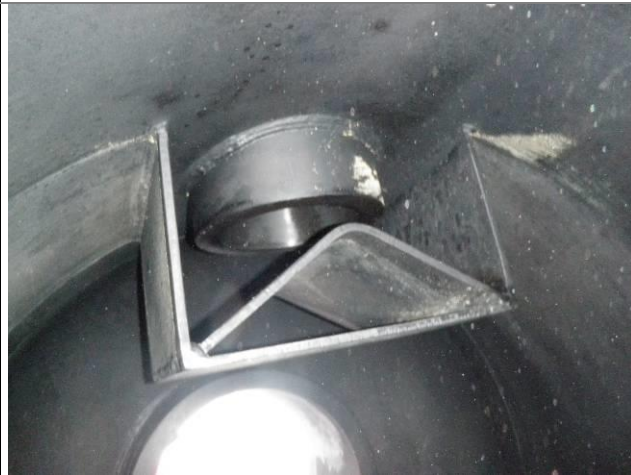
INLET NOZZLE DEFLECTION PLATES
